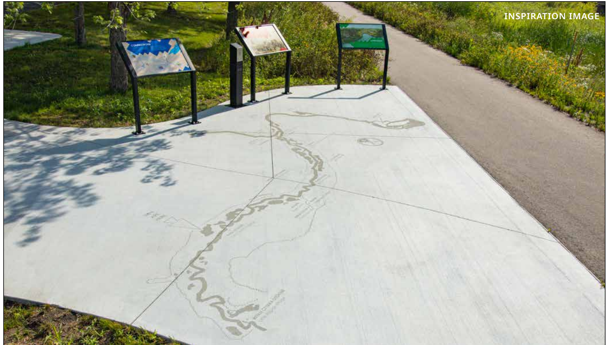
Example of concrete etching
